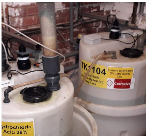
dBR8's reading through the plastic lid of a chemical tank.
